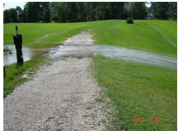
Photo 2: Embankment overtopping in June 2011.
