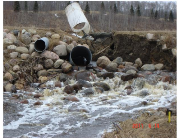
Photo 1: Embankment washout apparently due to culvert piping in April 2011.
