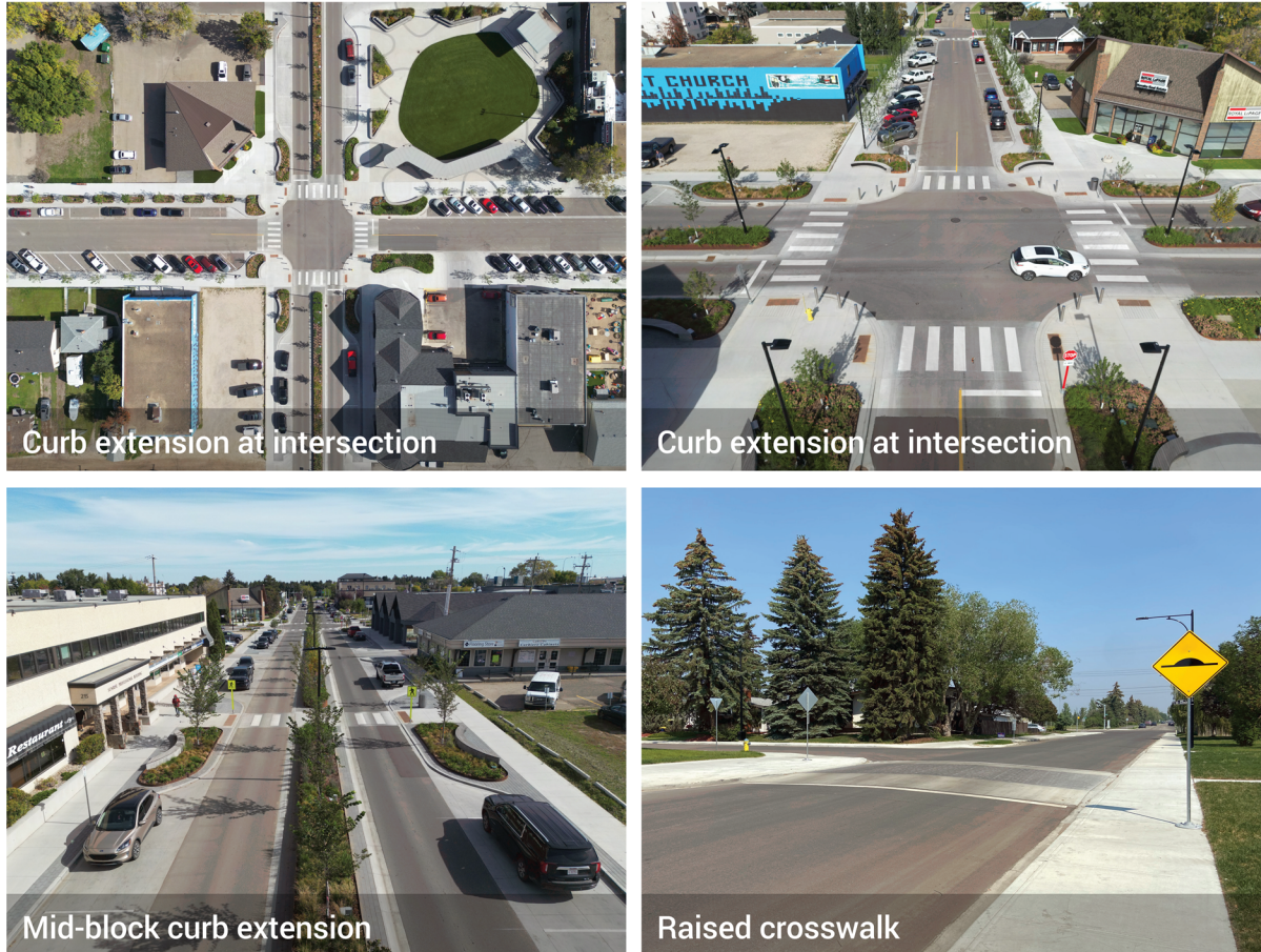
Figure 6.15 Traffic Calming Measure Examples
