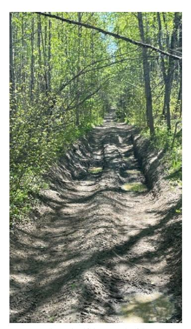
Figure 8: Typical cupped and failing seismic line following recreational use
