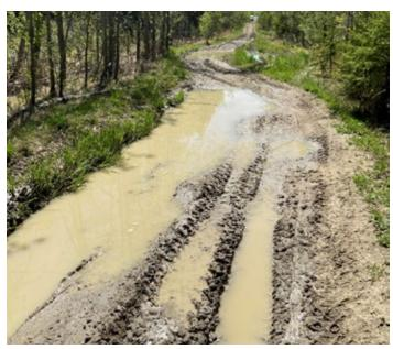
Figure 9: Typical cupped and failing seismic line following recreational use
